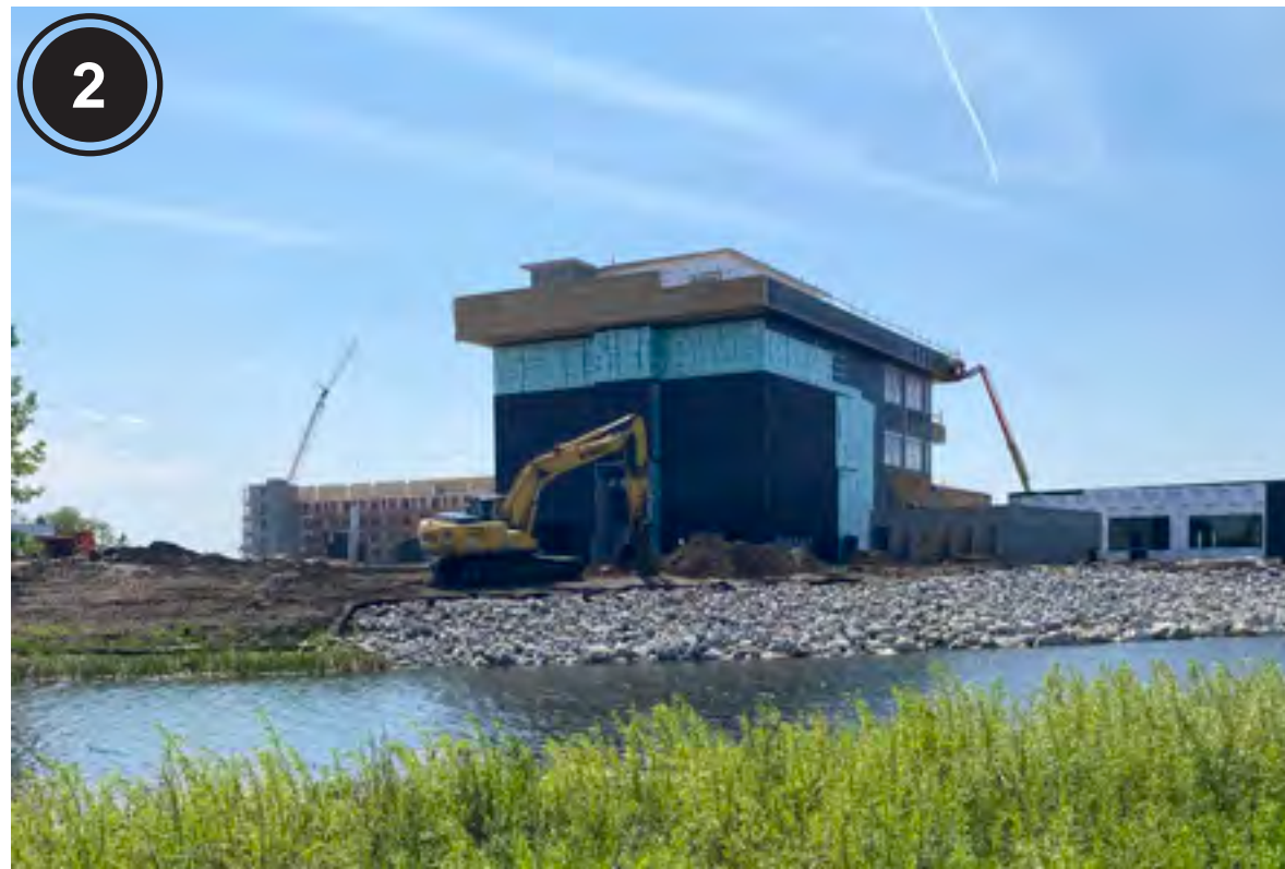
2 EXISTING SHORELINE HAS RECENTLY BEEN STABILIZED WITH RIP RAP
