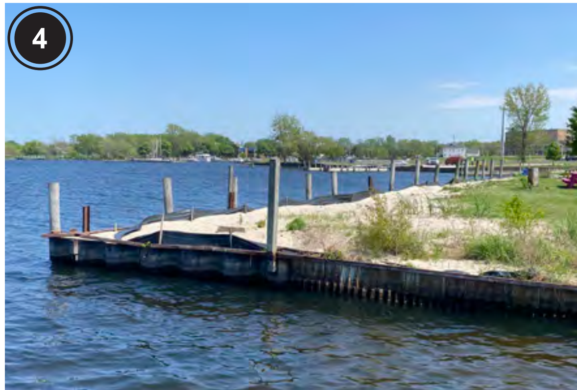
4 EXISTING SHEET PILE WALL
